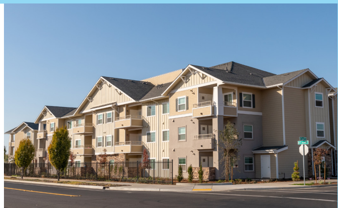
Bow Street Apartments – Elk Grove, CA.
