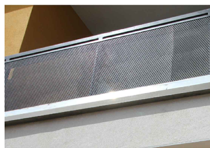
(7) METAL RAILING SYSTEM PERFORATED METAL SCREEN
